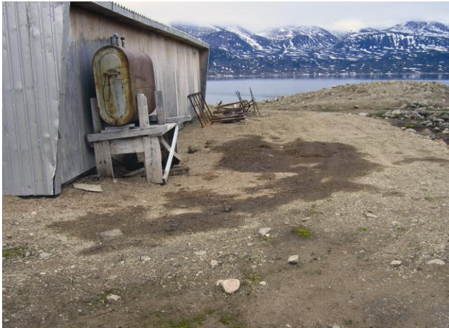
Unstable fuel tank on wooden stand and oil staining on ground.
