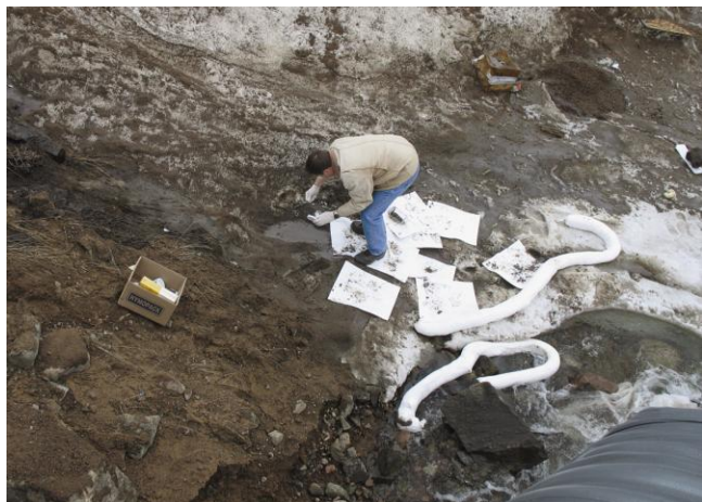
Recovering pooled oil using absorbent pads and booms.
