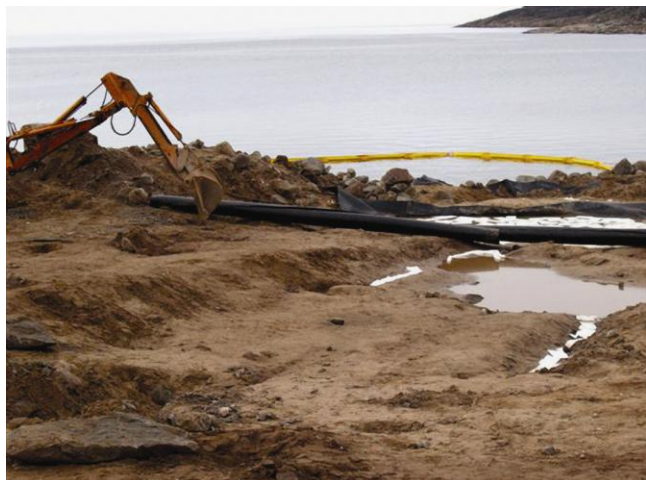
Installing a containment berm and liner near the ocean.
