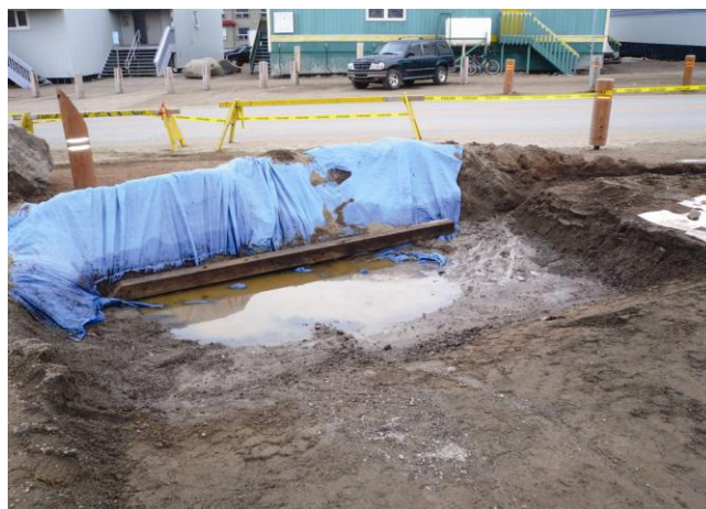
Excavated contaminated soil.
