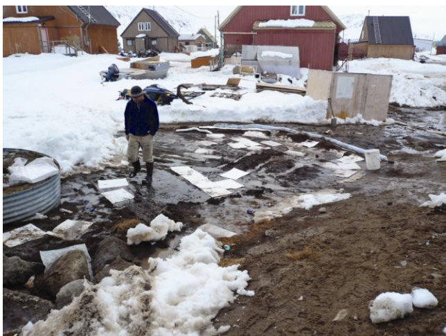
Cleanup of spring melt water using a temporary dyke and absorbent pads.
