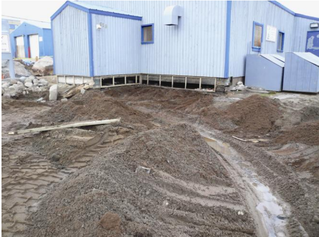
Excavation to remove contaminated soil near building foundation.
